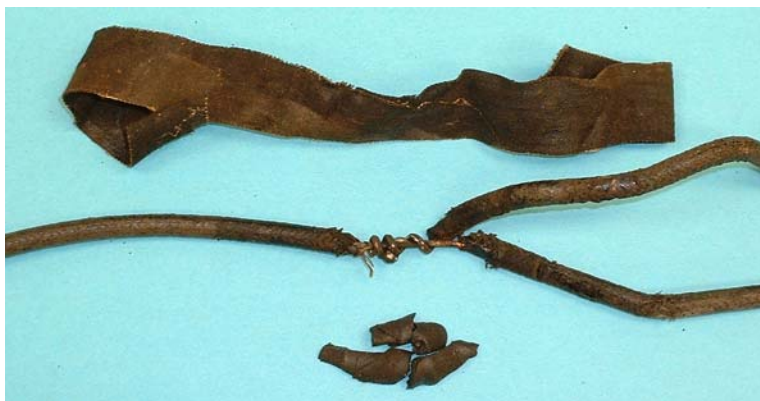
Fig. 11 – Soldered Splice with Friction Tape (top) over Rubber Tape (bottom)
